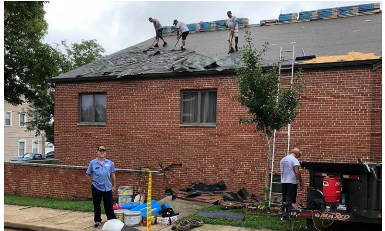
Mike Hill watches the roofing process
